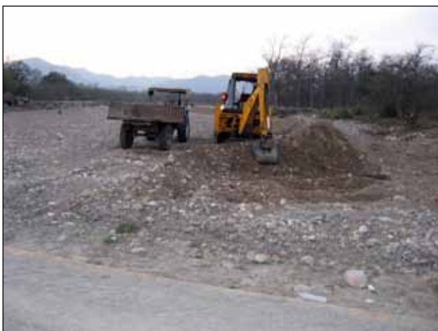
Figure 4. Construction of temporary car parking.
