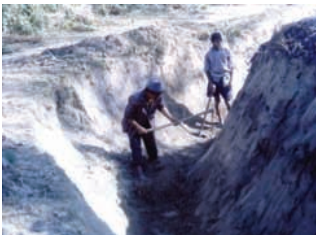
Figure 1. Elephant proof trench digging.
